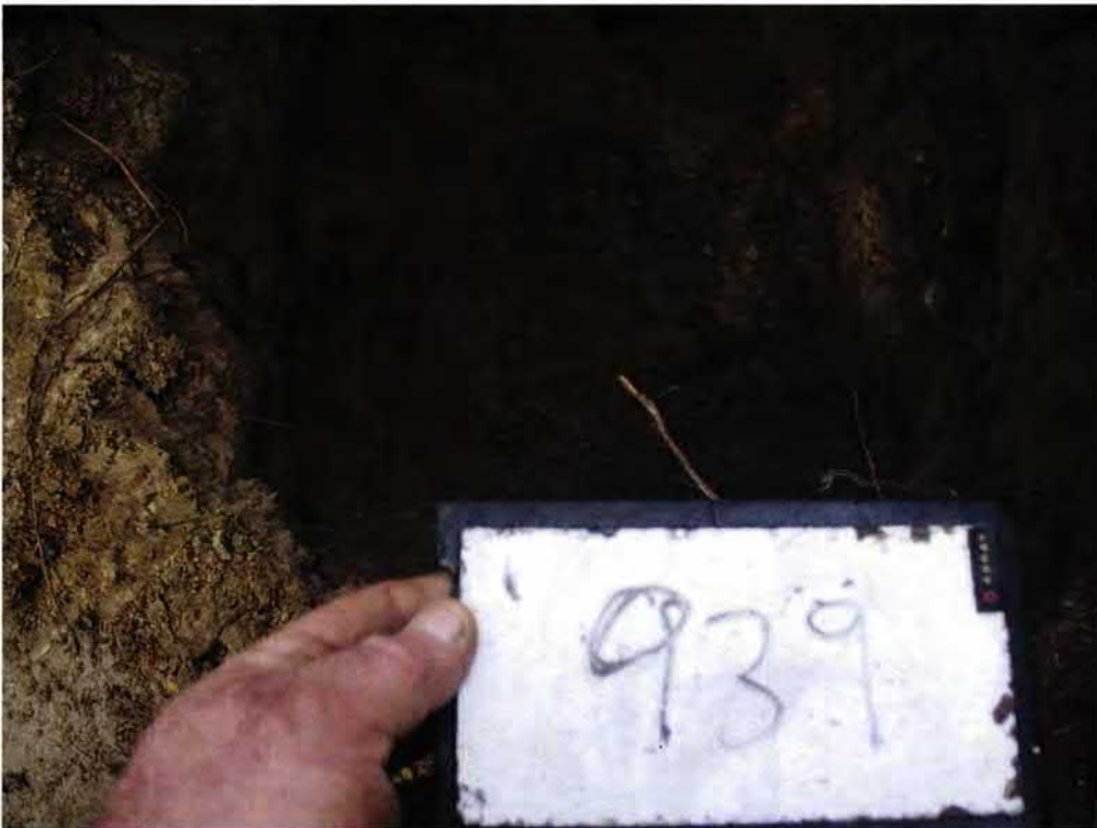
Picture 2: UST 939Albacore excavation.
